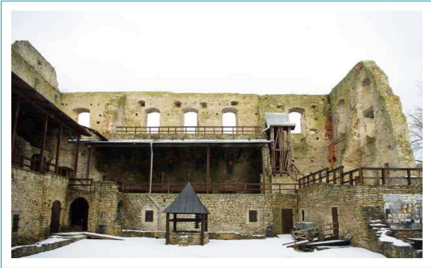
*Image No. 3, Before the works. In 2014, the castle walls and later additions were in emergency condition. Photo SALM.*
