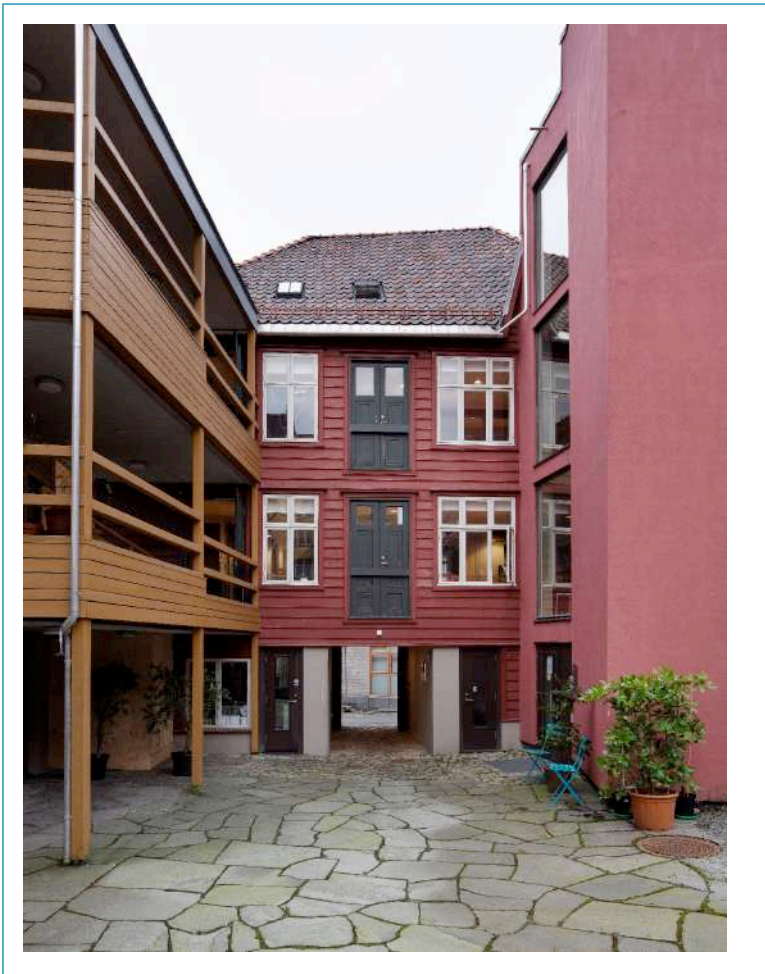
No. 15 The Agency for Cultural Heritage Management in Bergen façade from the backyard. Photo: Trond A. Isaksen, Directorate for Cultural Heritage
